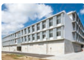
NII's Kashiwa Annex
